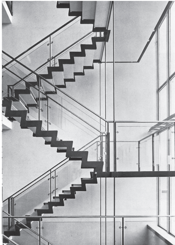
Figure 15. Arne Jacobsen, city hall in Rødovre, 1954-56. The suspended steel staircase in the main lobby facing a curtain wall, towards the back. Bloxham Zettersten, Nordiskt perspektiv på arkitektur , 342; photo: Strüwing.
