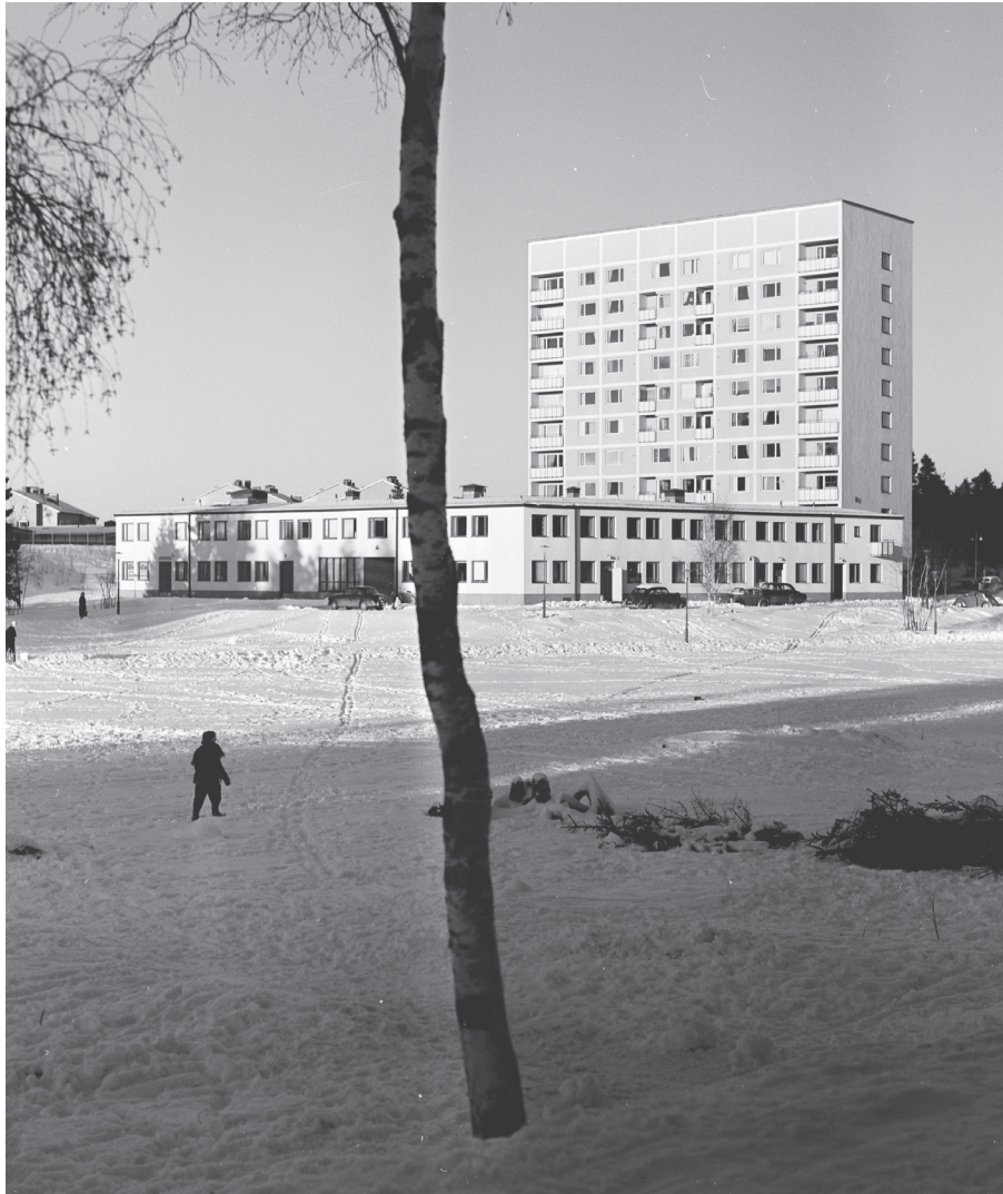
Figure 1. Stockholm suburb Bandhagen designed by Fred Forbat, Bengt Karlsson and Curt Strehlenert. Photo: Sune Sundahl, 1956. ArkDes collections.
