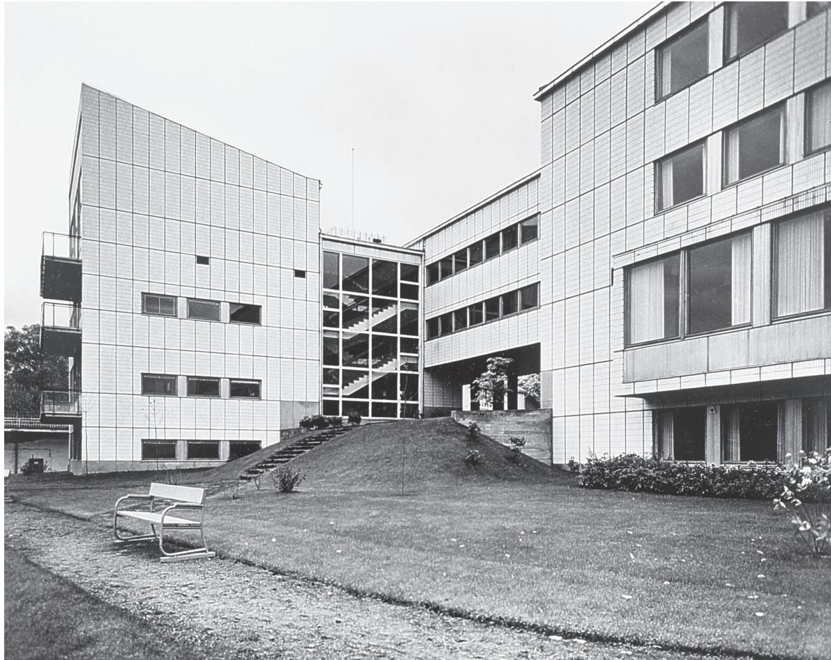
Figure 14. Risto-Veikko Luukkonen, municipal hall in Valkeakoski, photo showing the main staircase behind a glass panel façade, connecting the council chamber wing and the bridge element. Bloxham Zettersten, Nordiskt perspektiv på arkitektur , 326; Museum of Finnish Architecture.
